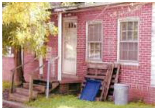
Camp Drive Building / CORA Entrance
